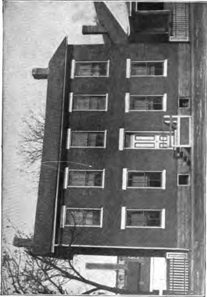
HAYES HOME AT DELAWARE, THE BIRTHPLACE OF RUTHERFORD BIRCHARD HAYES. The first brick dwelling-house in Delaware, Ohio; erected by the father of Rutherford Birchard Hayes, Captain Rutherford Hayes (1787-1822), prior to his death July 20, 1822.
